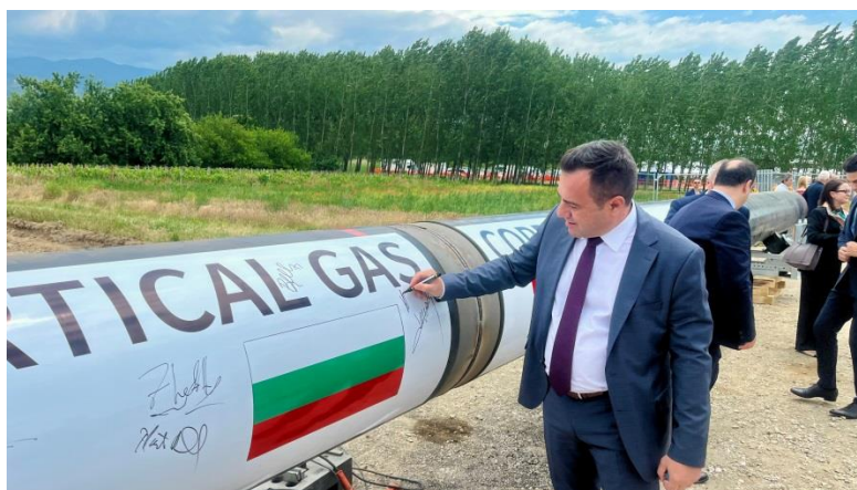
EWRC Chairman Plamen Mladenovski participated in the inspection of the Vertical Gas Corridor construction progress
